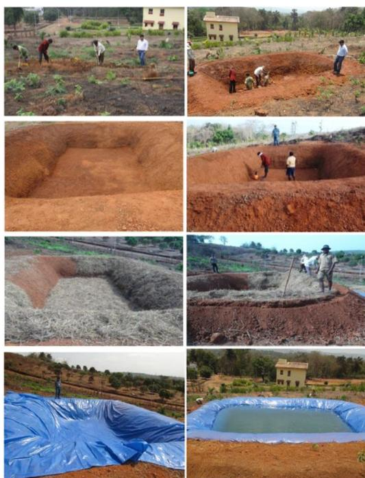
Figure 5, the various stages of Jalkund construction
