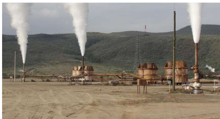
Figure 4. Emission (including  $H_2S$ ) from the discharge and flow testing wells at East Olkaria.
