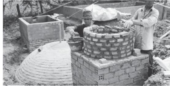
**Figure 5: Construction of biodigesters in Cambodia through the National Biodigester Program (NBP, n. d.)**
