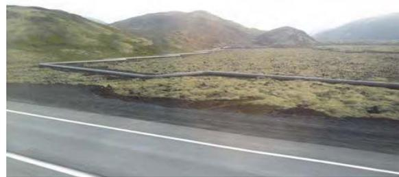
Fig. 7 Above: Geothermal plant at Nesjavellir. Below: Part of 23 km pipe for hot water, from Nesjavellir to Reykjavik.
